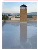
One component liquid waterproofing composition, after polymerization gives an elastomeric, coldapplied polyurethane membrane.
